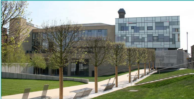
Barnsley Civic Centre, UK Glass Wagener supplied low-E glass and 400 sqm Vacurex panels (U-value 0,31 W/m²K)
