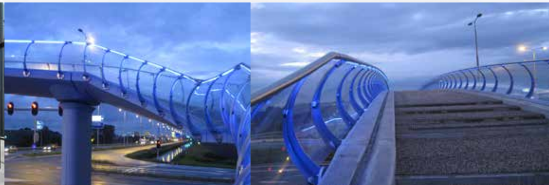
Pedestrian bridge | Bleiswijk | 150 m 2 | Fini Curve VSG (laminated glass) 66.4 / float
